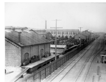
Ca. 1908 photograph of railroad tracks and buildings in South Tacoma including some of the Northern Pacific Shop buildings. Amzie D. Browning Collection BROWNING-079. Courtesy Tacoma Public Library.
