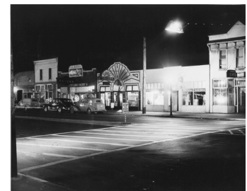
A marked and lighted crosswalk on South Tacoma Way as photographed at night on May 29, 1949. Richards Studio D42516. Courtesy Tacoma Public Library.
